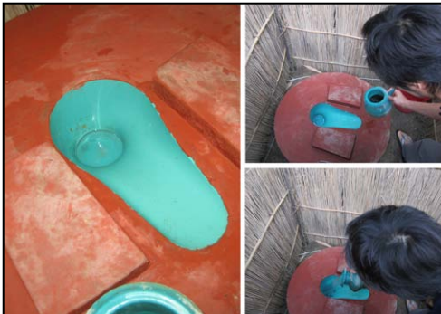
This SaTo toilet pan, short for Safe Toilet, was developed by American Standard to reduce disease transmission in Bangladesh by sealing off pit latrines from the open air by employing basic mechanical and water seals.
