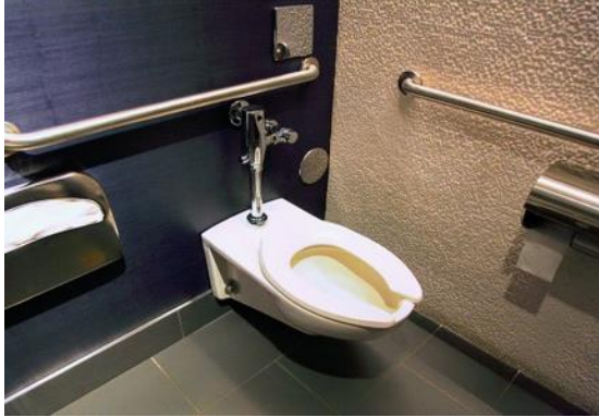
Both the SunTrust Club and the Delta Sky360 Club provide a clean, comfortable experience for their club-level ticket holders, with the high-performance American Standard AFWall Millennium FloWise toilet and manual flush valve that consume only 1.28 gpf.
