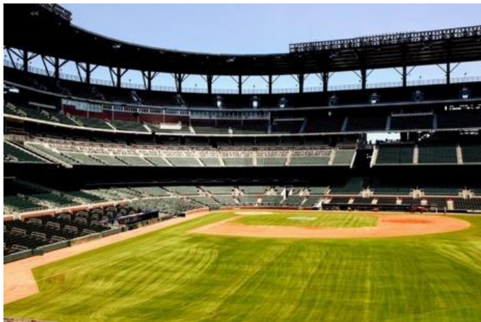
American Standard, provided faucets, sinks, toilets, urinals and showerheads to outfit the restrooms and locker rooms in the new 41,000 seat SunTrust Park.
