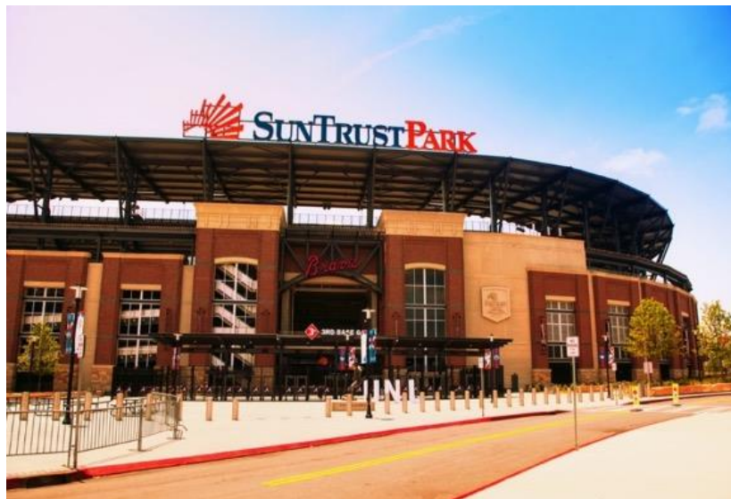
In 2017, Major League Baseball's Atlanta Braves moved into the newly constructed SunTrust Park. The Braves partnered with American Standard to install fixtures and fittings in all bathrooms and locker rooms throughout the building.
