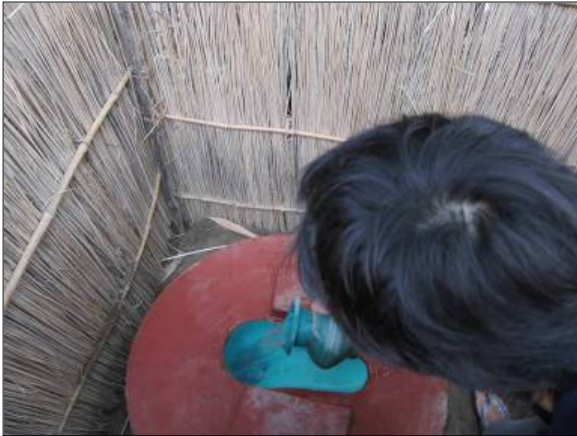
Users “flush” into pit latrines using a container called a “bodna.” American Standard’s goal in creating SaTo was a solution that fit both local customs and typical pricing, in order to encourage widespread adoption of a safer alternative.
